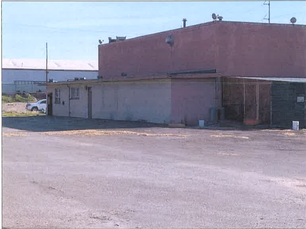
Westerly façade looking northeast.
