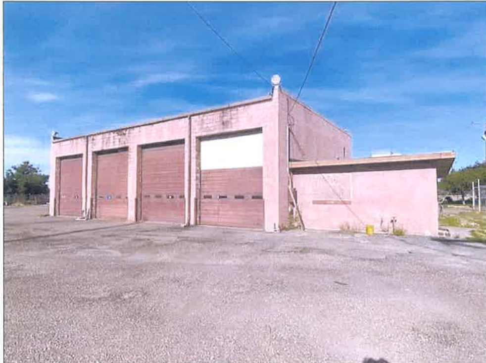
Easterly façade looking west.
