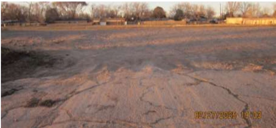
Staff Photo at end of Riley Drive's pavement ending at a 20' wide east/west alley right-of-way contiguous to Property's south boundary; looking toward houses in North Plains Park 3 Subdivision separated from Property's north boundary by alley right-of-way.
