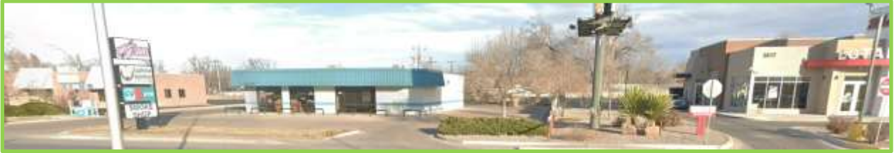
Image Date 12/24 Google Earth Photo looking east toward Commercial Building at 3107 N Main Street showing Blake's Lotaburger adjacent to the south and The Ivory Brunch House adjacent to the north.
