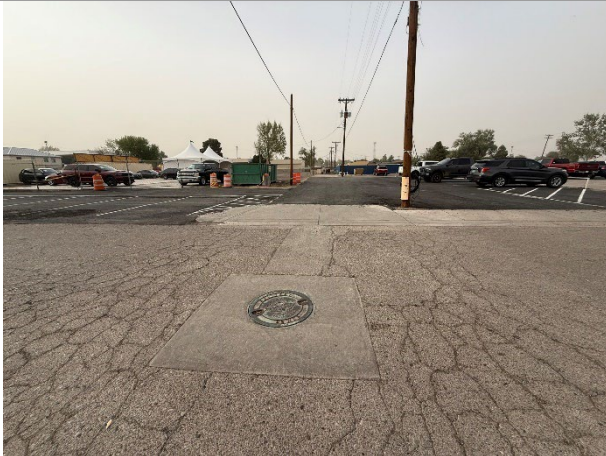
ALLEYWAY PORTION OF SUBJECT SITE, LOOKING SOUTH ACROSS 9 TH STREET
