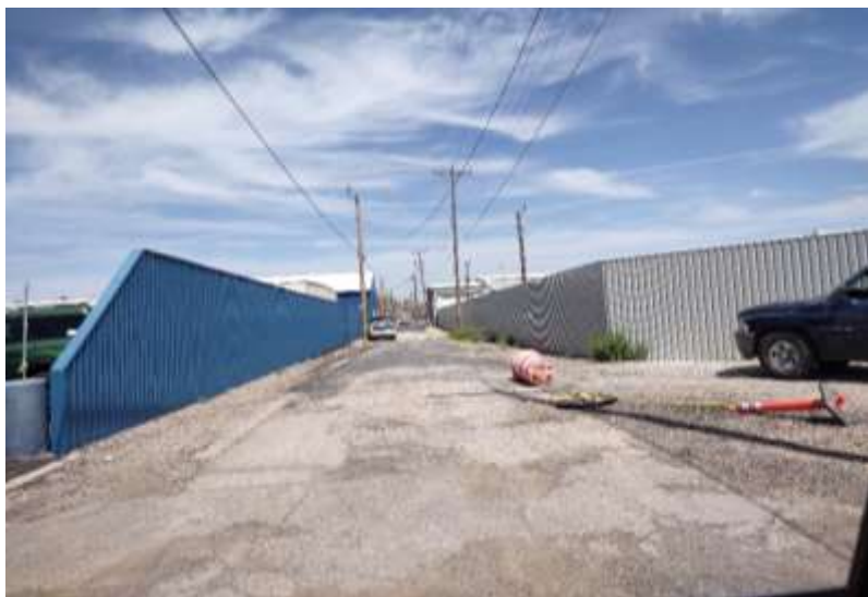
Looking North from 8 th Street at Alley located between Rhoads Company on the east and Roswell Ford on the west.
