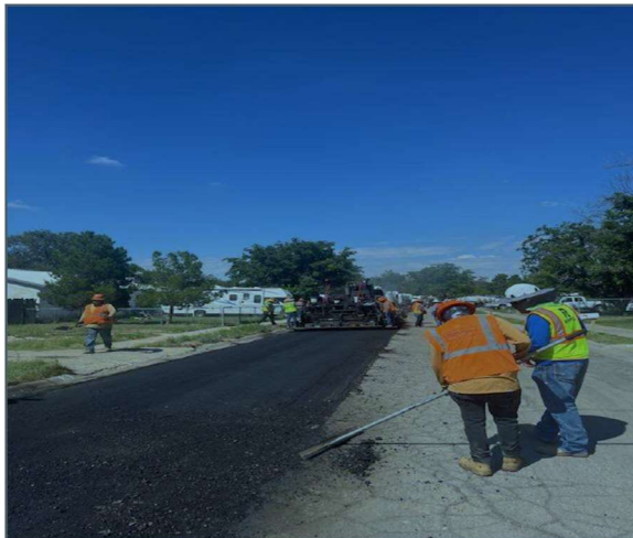
Example of Hot Recycling Process
