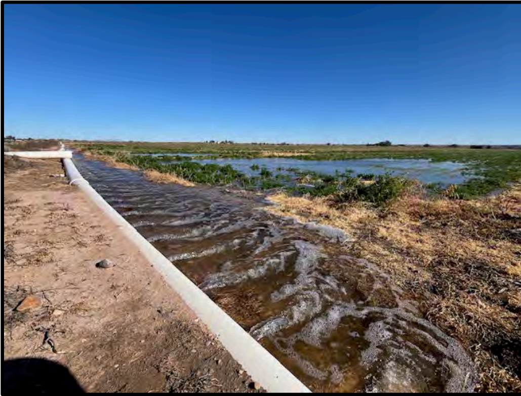
Subject Irrigation System
