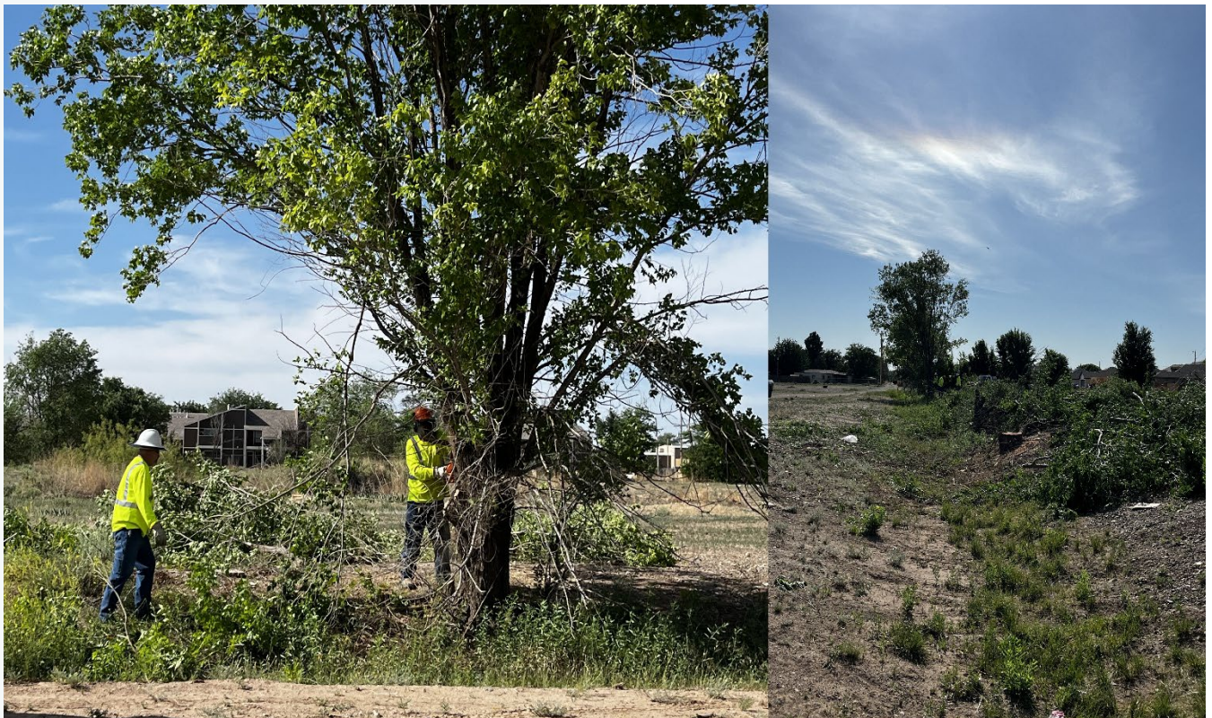
Heath and Jerry work to remove trees posing a danger or obstructing views and access.
