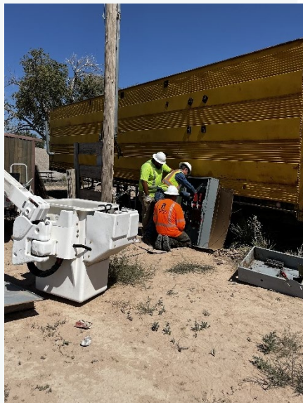
Clifford and the Special Electronics Team replacing the 400 amp disconnect switch at the city crusher site. Thank you, Special Electronics!
