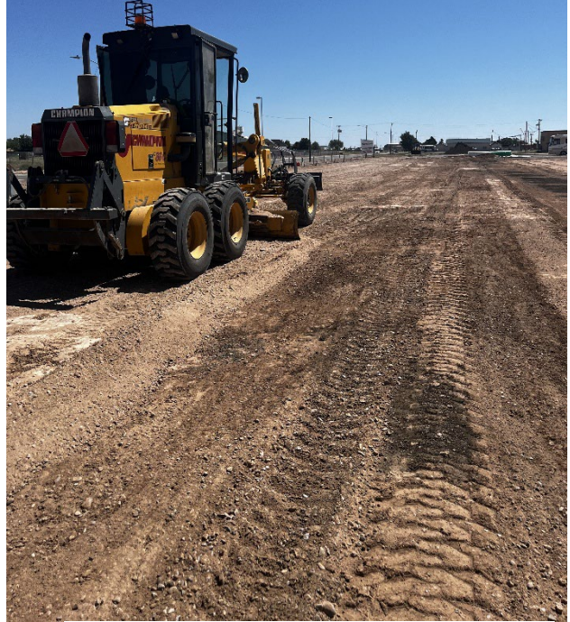
Ongoing work for the NCAR parking and RV lot
