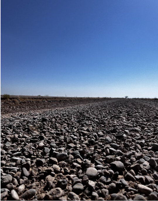
Regraded access road for residents behind the base for the air races
