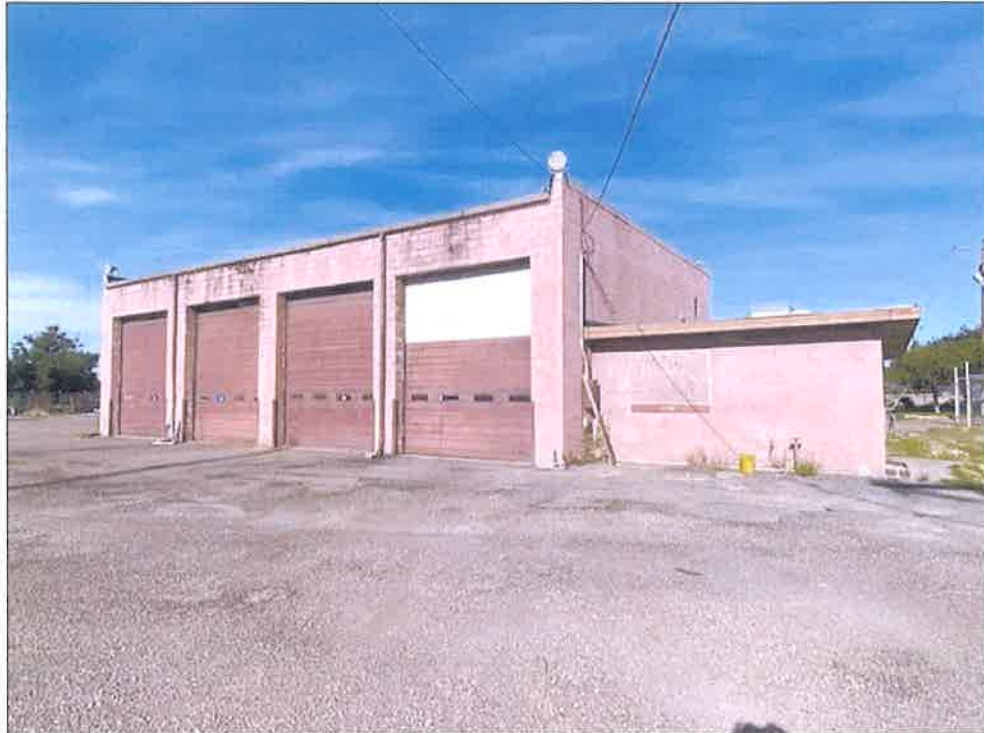
Easterly façade looking west.
