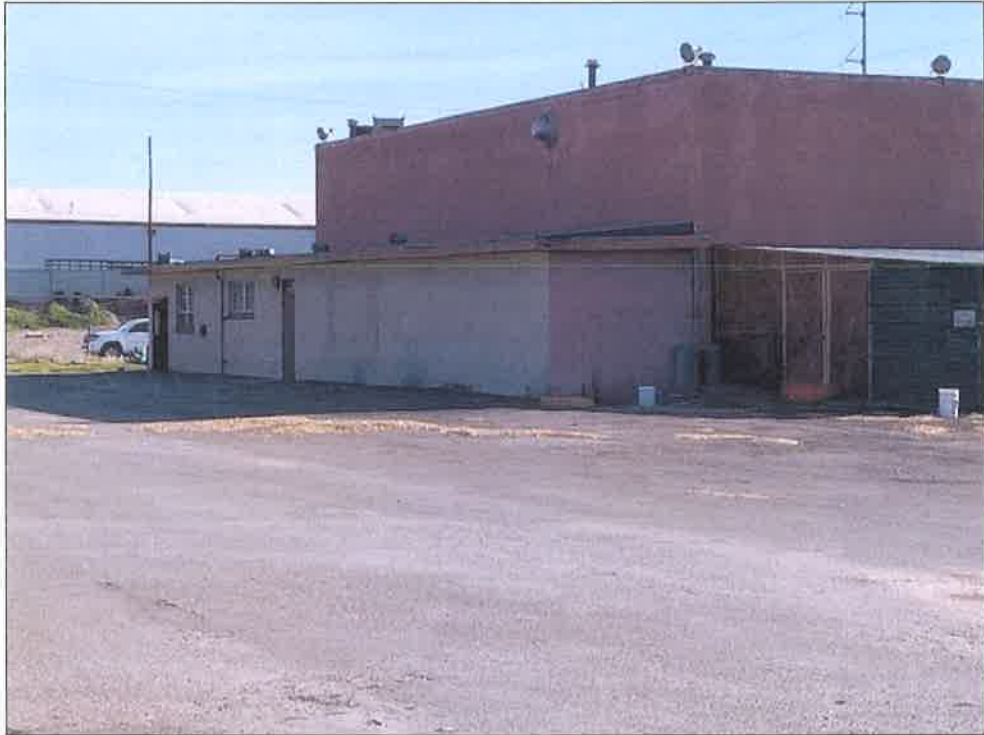
Westerly façade looking northeast.
