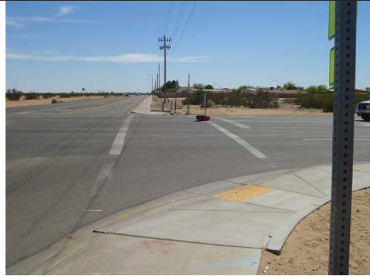
18. NWC Ped ramps and crosswalk
