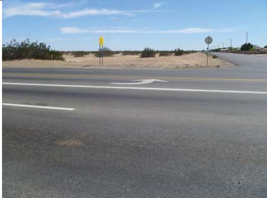
5. NEC looking south
