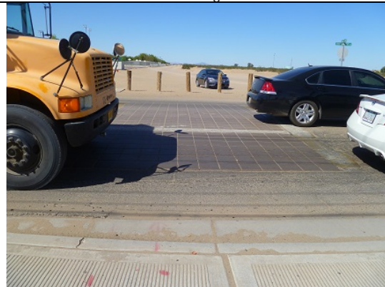
16. Ped ramp, crosswalk west of 1 st close-up
