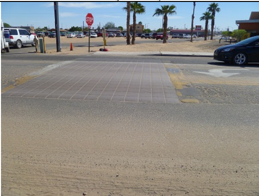
15. Ped ramp, crosswalk west of 1 st close-up looking south
