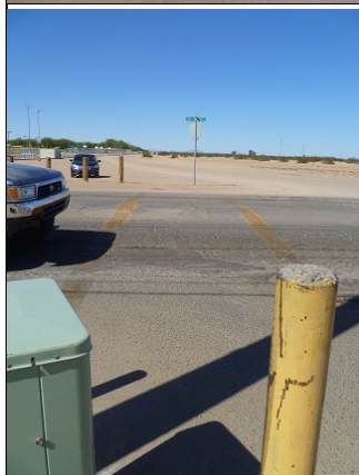
23. SWC 1 st crosswalk to north Access
