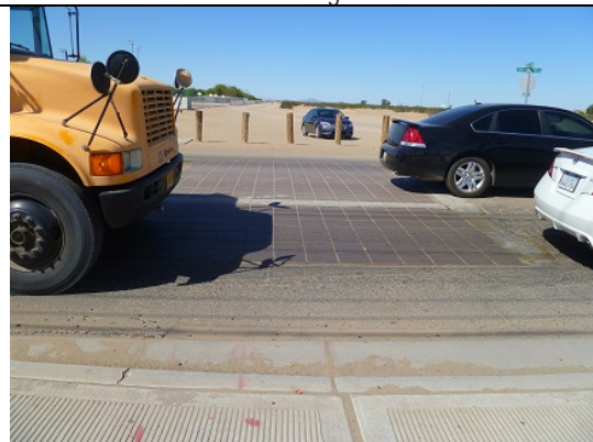
16. Ped ramp, crosswalk west of 1 st close-up
