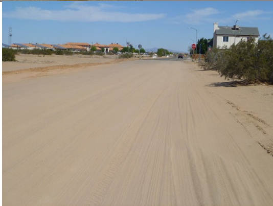
29. Union Access looking east
