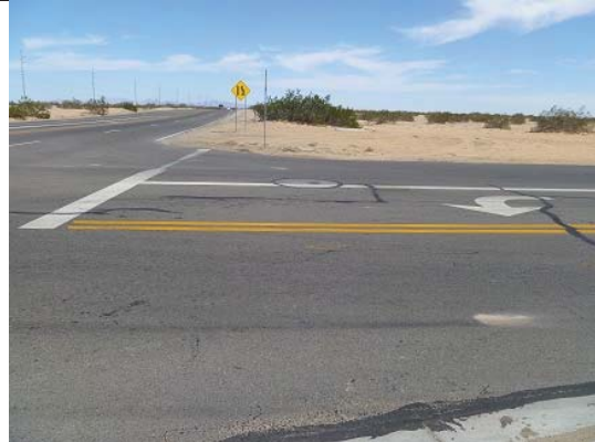
28. SWC looking east 2
