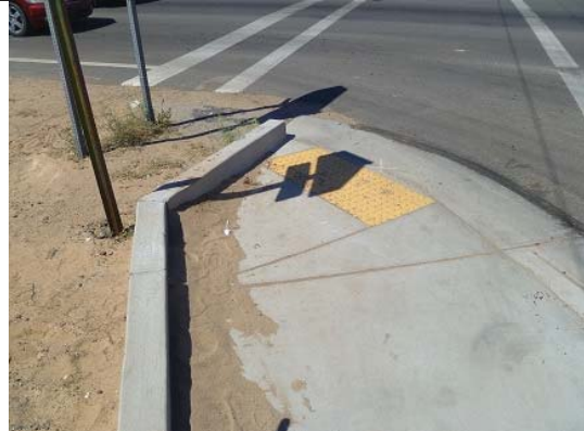
30. SWC Ped Ramp
