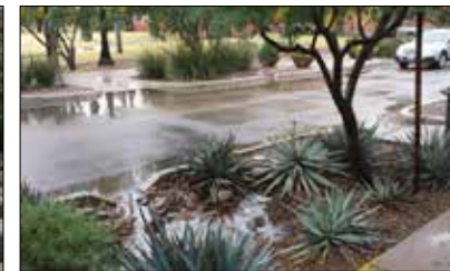
Benefits of Bulbouts include reduced pedestrian crossing distances, traffic calming, water harvesting, green infrastructure, treats runoff and irrigates plants
