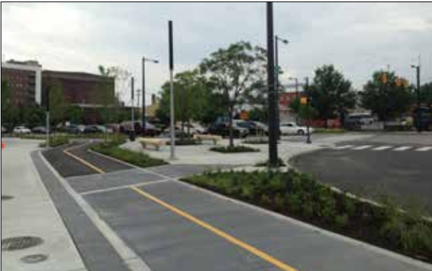
Cycle Track helps improve safety and reduce stress, encouraging residents to take up bicycling
