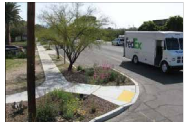
Figure 26. Examples of green infrastructure in arid communities that provide stormwater runoff management and treatment along streets.
