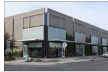
Buildings at street provide interest and convenient access to pedestrians
