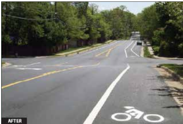
Road Diet technique can be applied to provide space for improving pedestrian and bicycle facilities along existing roadways
