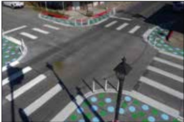
Paint/Planter/Bollards can be used to create identity/increase pedestrian comfort
