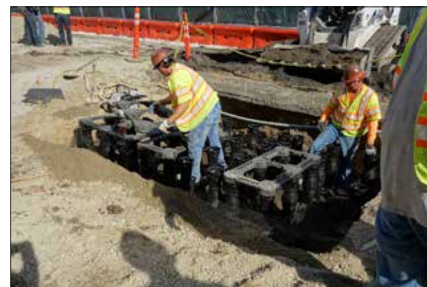
Figure 25. Examples of Green Infrastructure measures that can be used to manage and infiltrate stormwater runoff along streets or underground. Top: Rain Garden Middle: Infiltration Chambers Bottom: Modular pavement cell system
