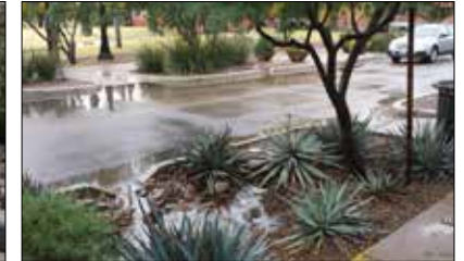
Benefits of Bulbouts include reduced pedestrian crossing distances, traffic calming, water harvesting, green infrastructure, treats runoff and irrigates plants
