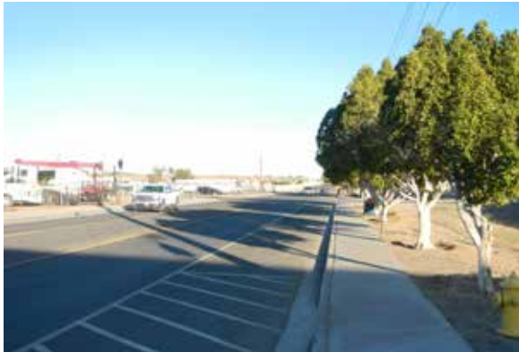
Urtzuastegui Street Existing Condition (Before)
