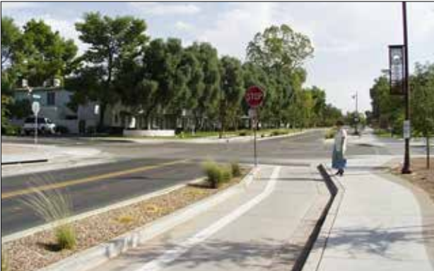
Buffered Bike lane helps improve safety and reduce stress, encouraging residents to take up bicycling
