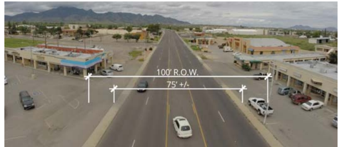
Fry Boulevard showing city ROW and roadway.
