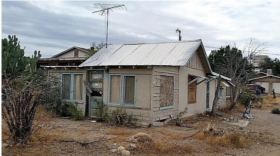
Property has dilapidated windows and doors and unclear walkways
