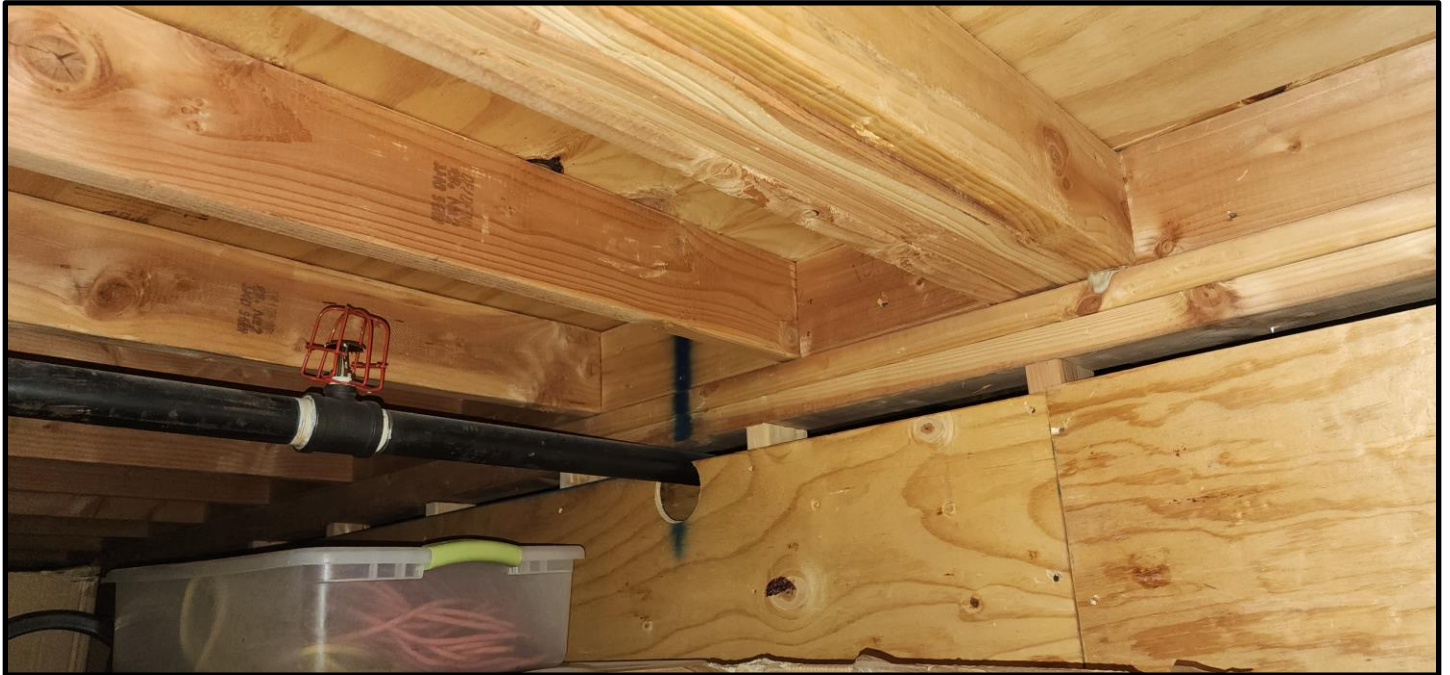
Sub floor in stage area
