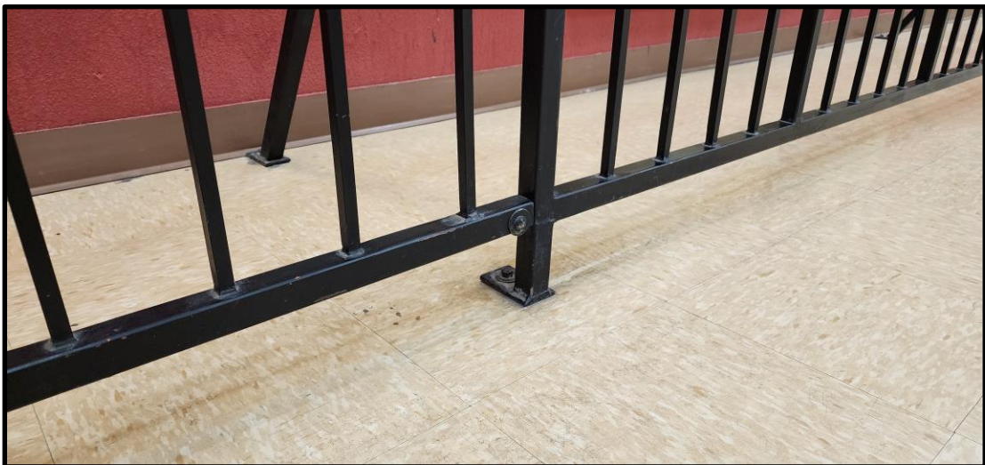
Main Floor Rails 2
