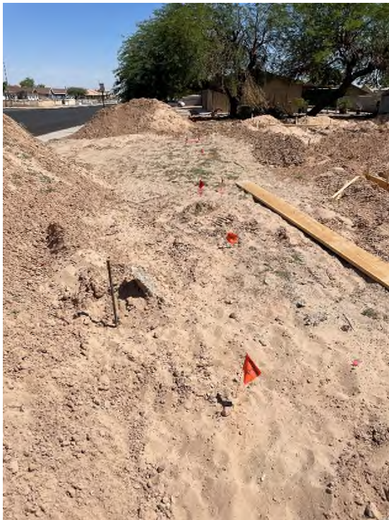
West side of property looking north. (Property corner location shown)
