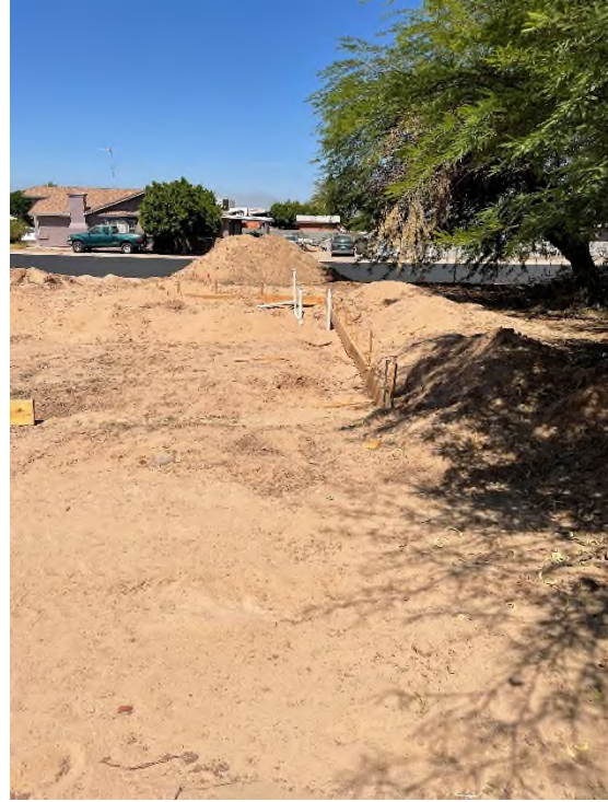
North side of property looking west.
