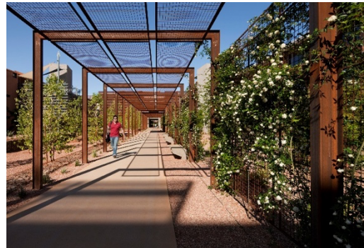
Example of a shade structure
