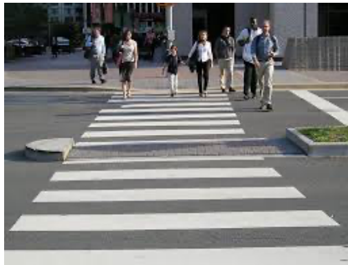
High visibility markings
