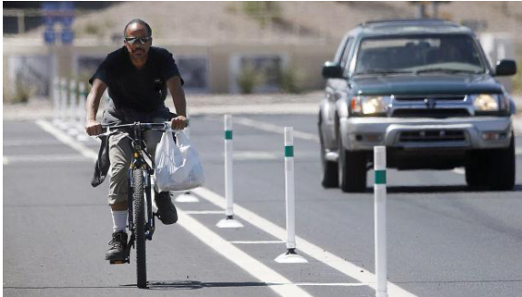
Protected bike lane with pavement marking buffer and vertical delineators.
