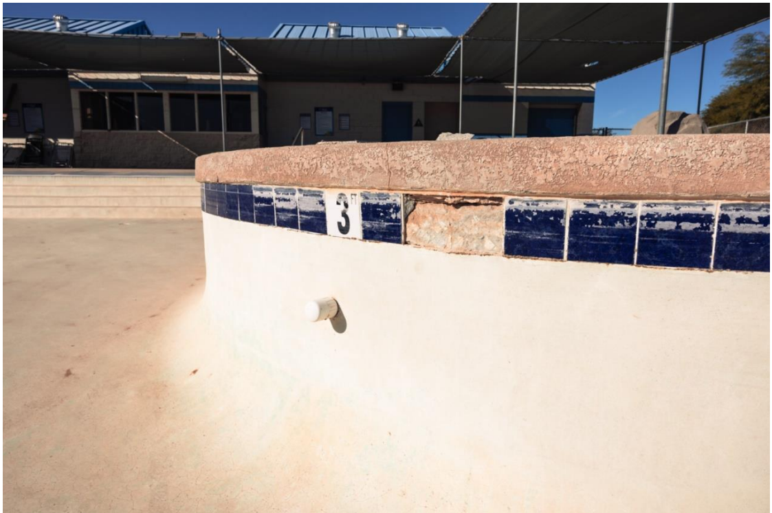
Pool Interior Tiles
