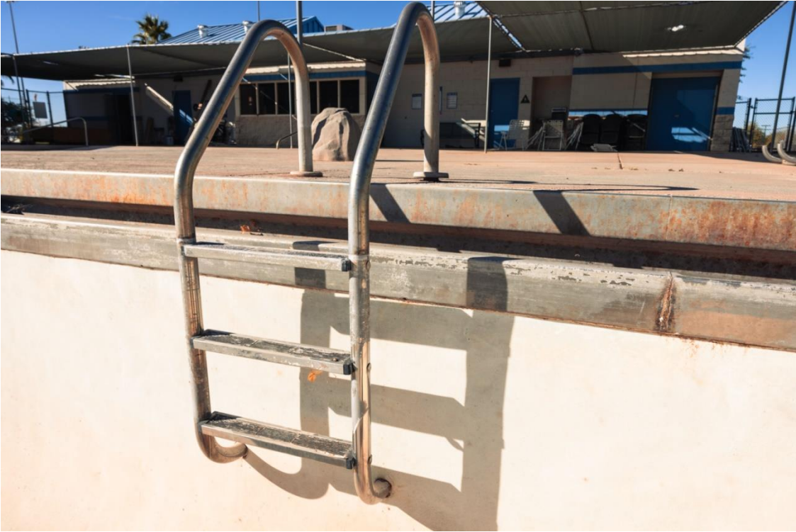
Pool Stairs and Gutter
