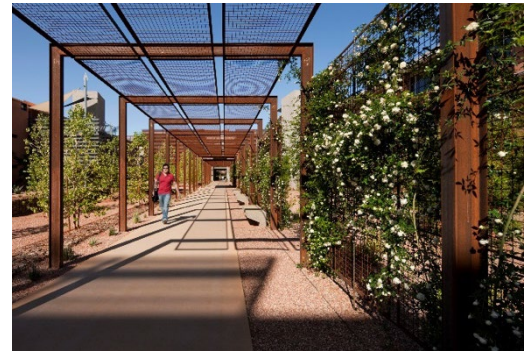
Example of a shade structure
