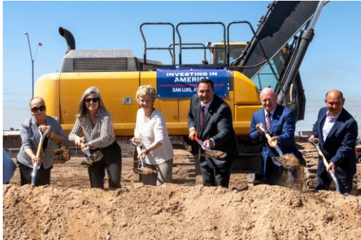
San Luis I Port of Entry Development: Overview of phased construction and IGA for cost-sharing improvements.
