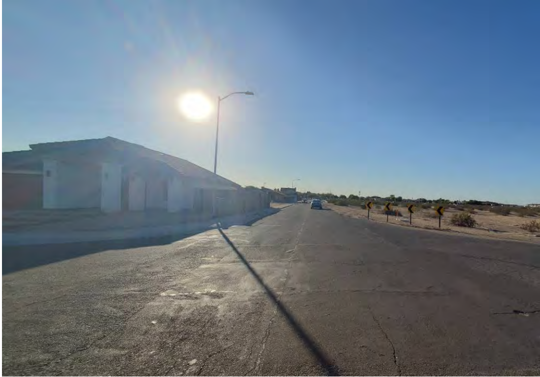
West Along Union Street, Subject Site at Right
