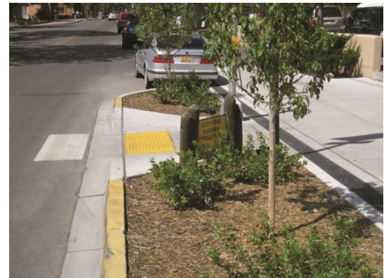
Example of curb extension that also provides additional landscaping in the streetscape.
