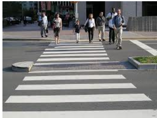
High visibility markings
