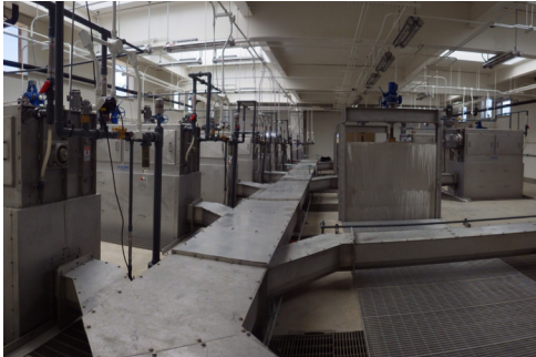
Dual stage screening with a common sluice shared by all screens and disposing into 3 washing compactors
