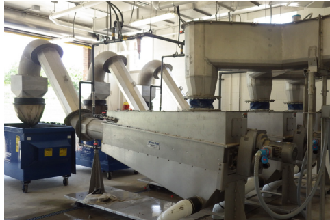
Dual stage screening with a common sluice shared by all screens and disposing into 3 washing compactors
