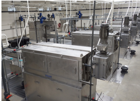
Right angle drive creates more open space around the screens
