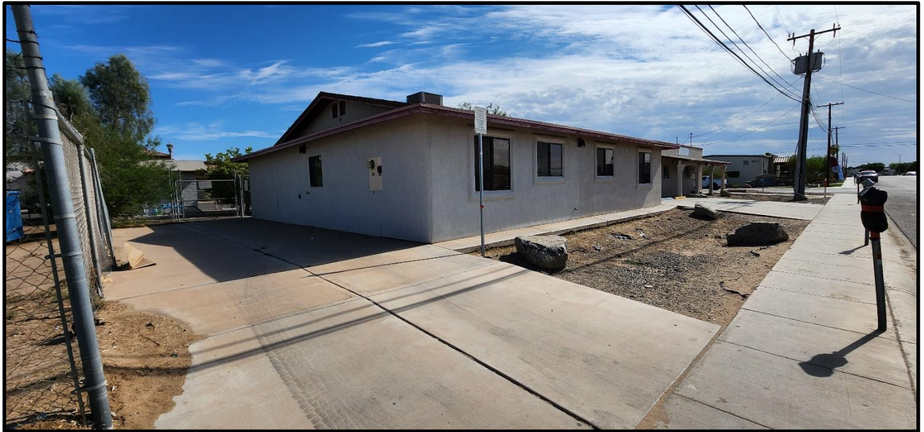
Exterior of Building
