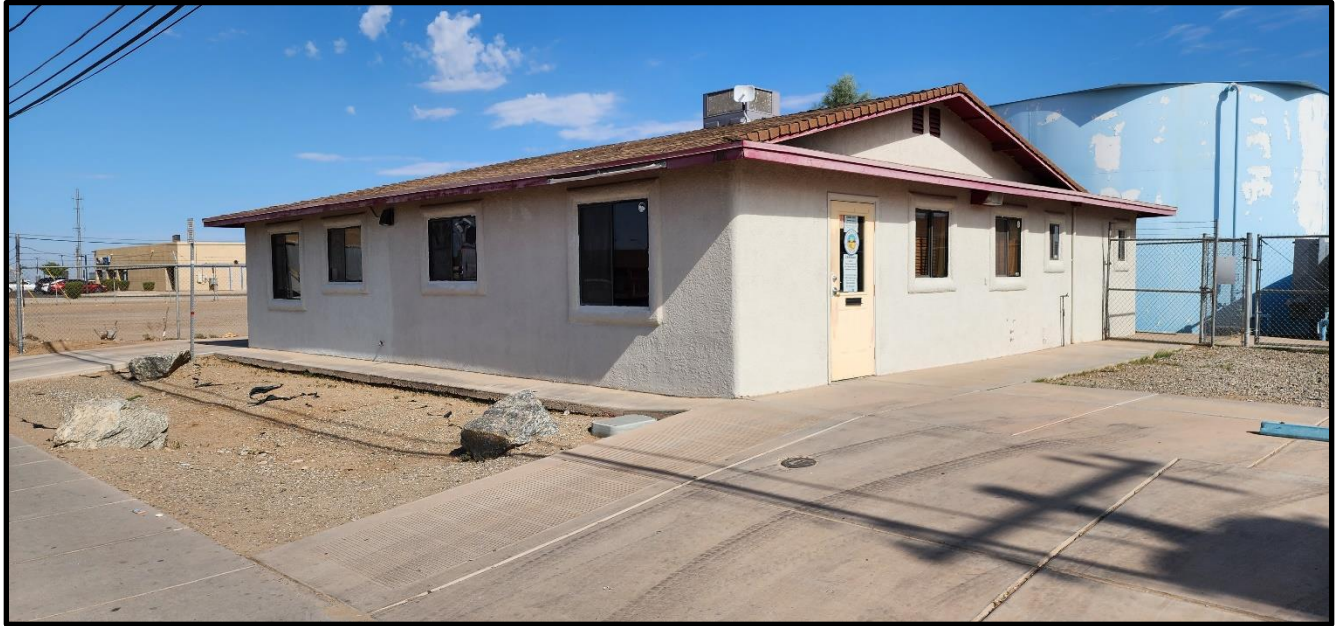
Exterior of Building
