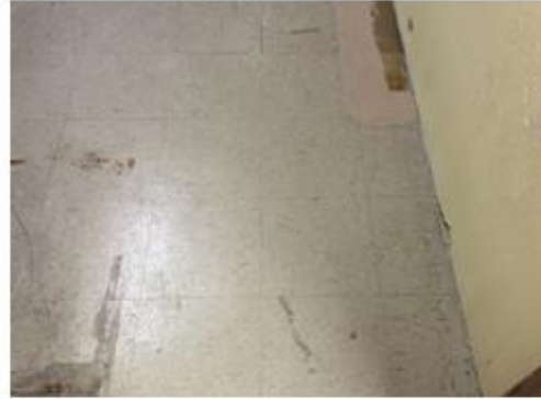
Encapsulation of Asbestos
