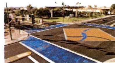
Example of an artistic crosswalk that reflects the character of the district.
