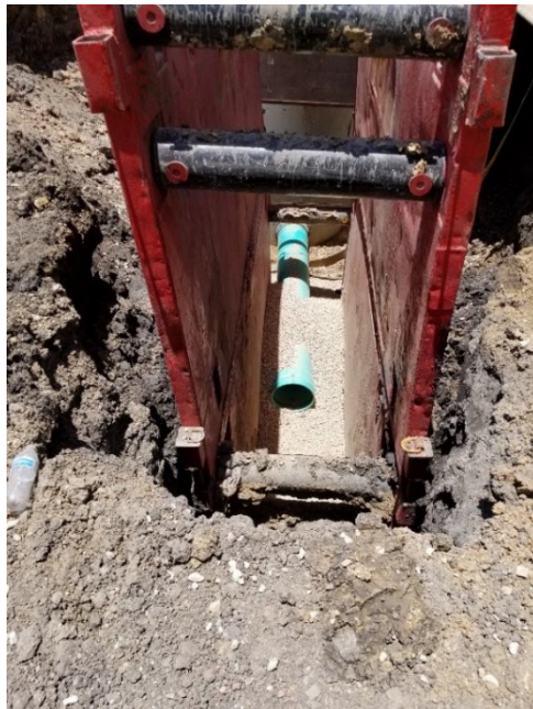
Starting Pipe Installation
