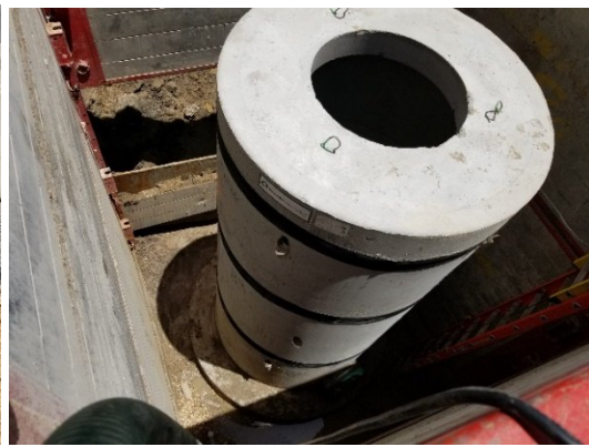
First New Manhole
