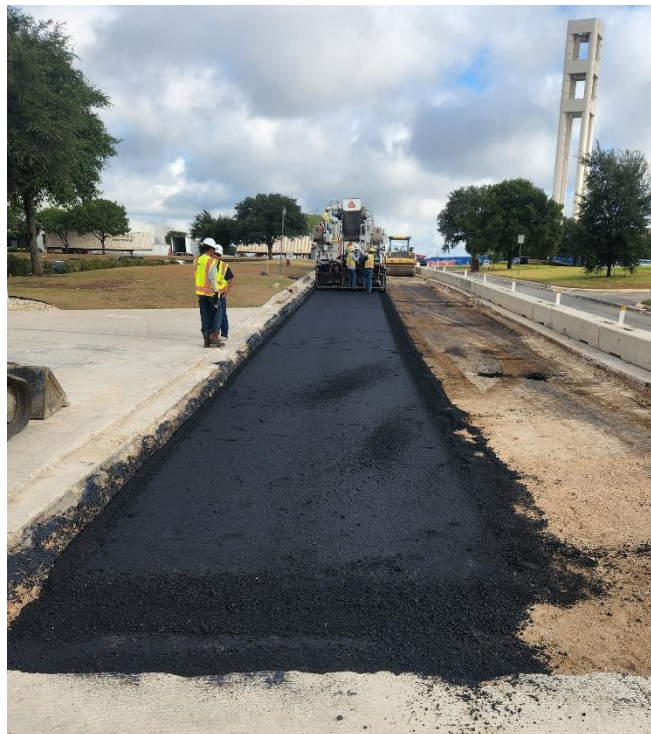
First Layer of Pavement
