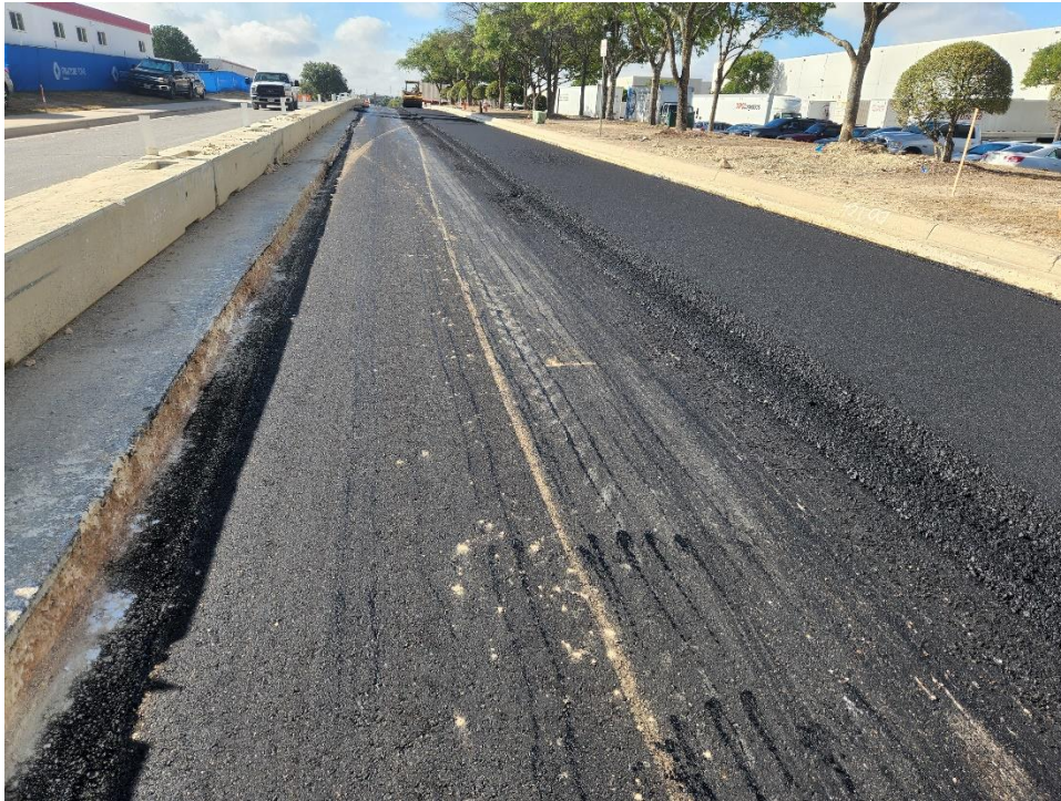
Second Layer of Pavement
