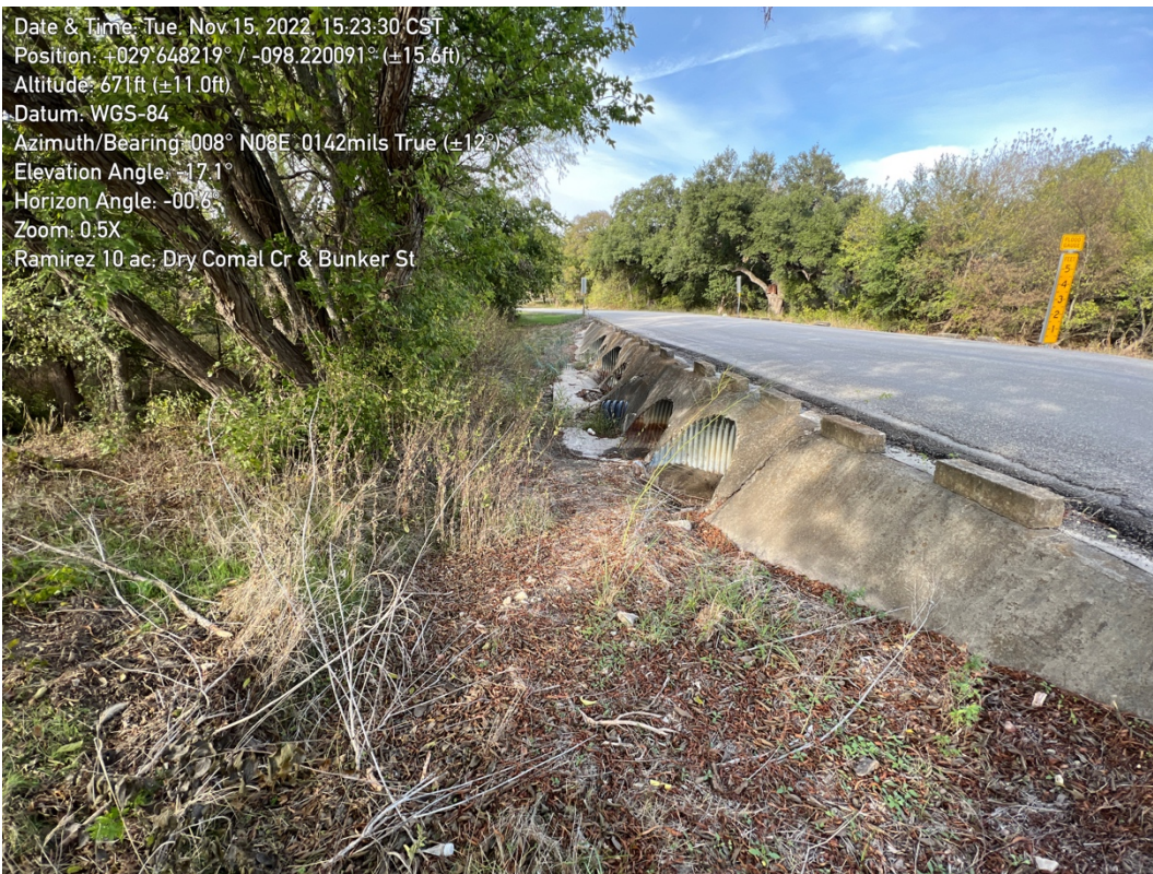
Photo 6. Bunker Street crossing of Dry Comal Creek (subject property on left).
