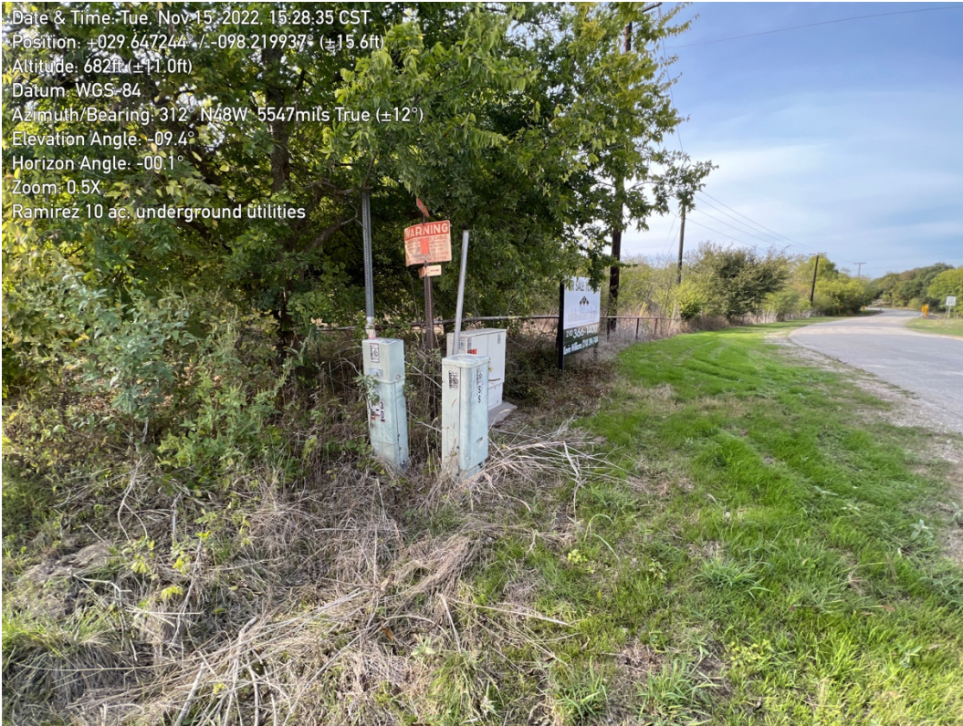
Photo 5. Underground utilities at southeast corner of subject property (Bunker Street on right).
