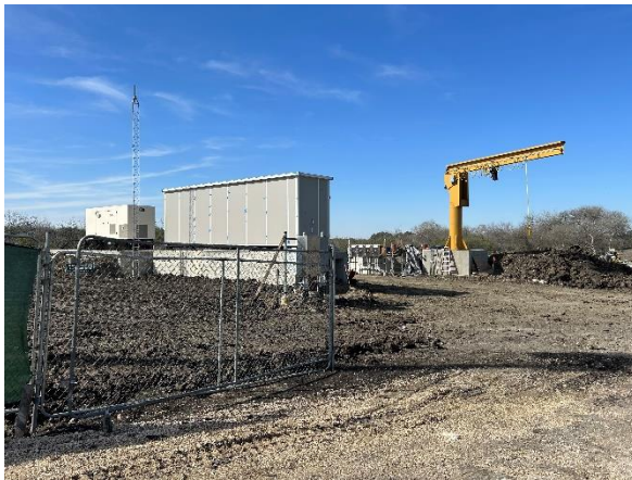
View of lift station site from IH 10
