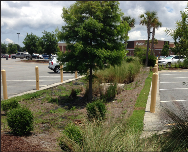
Parking Lot Drainage Swale
