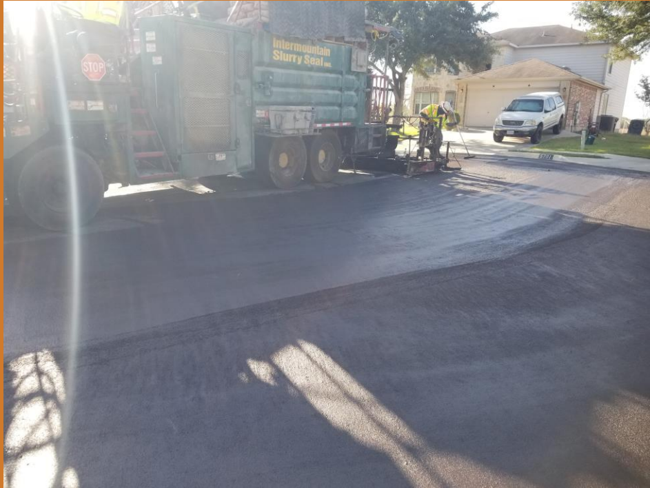
Slurry Seal/ Micropaving
