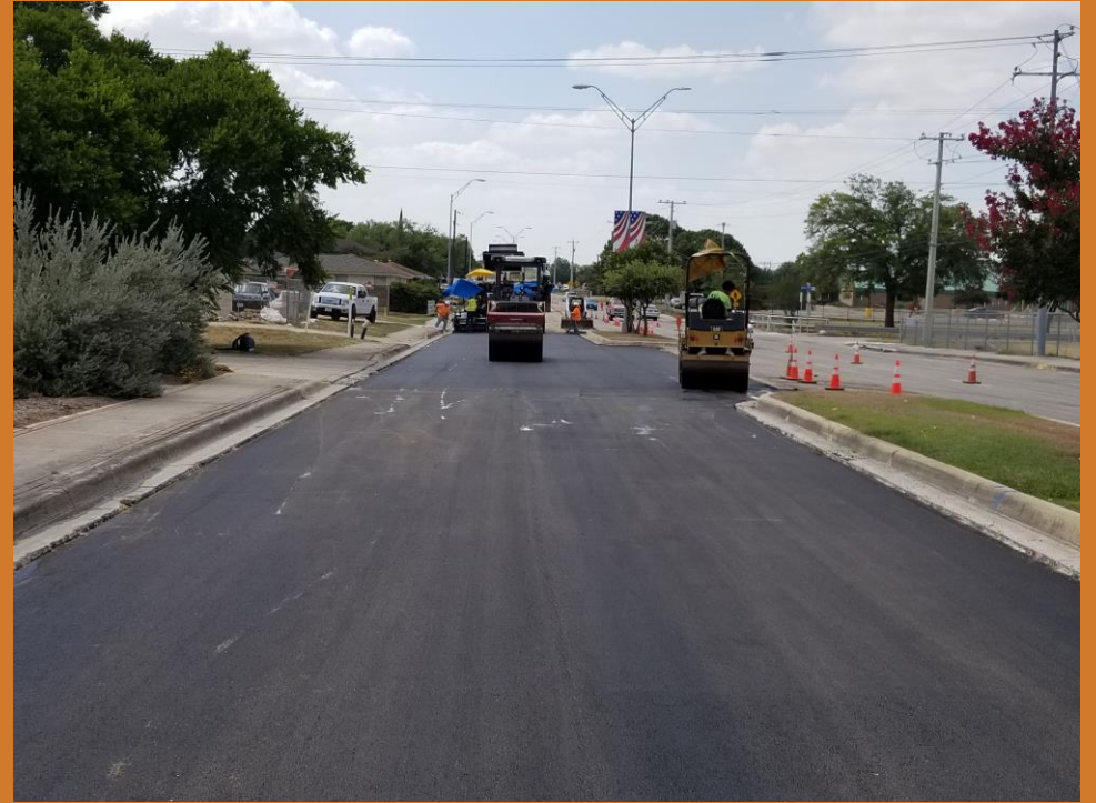
Mill and Overlay
