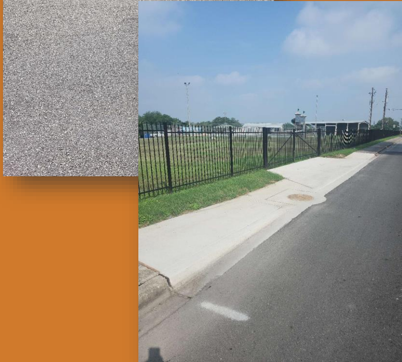
Concrete curb and sidewalk repairs.
