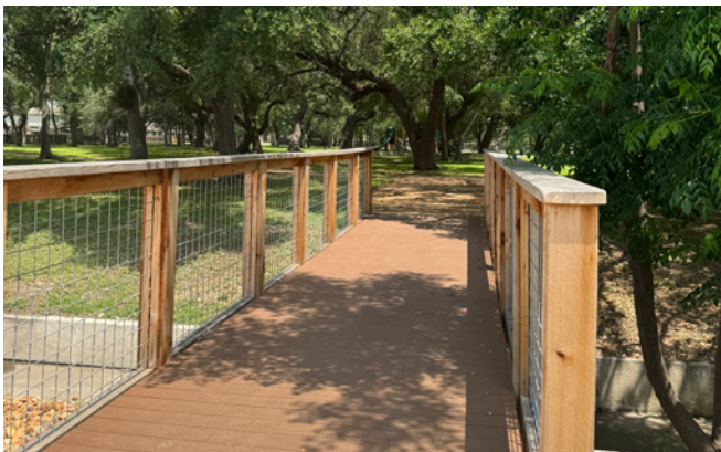
Bridge Crossing at Heritage Oaks Park
