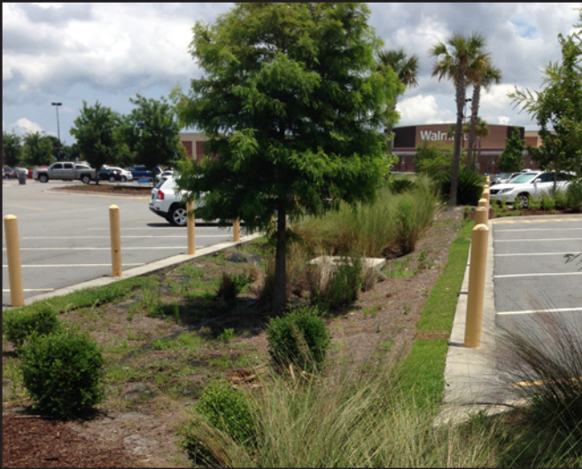
Parking Lot Drainage Swale
