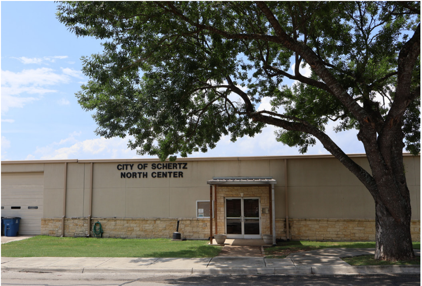
Existing Conditions of the North Center
