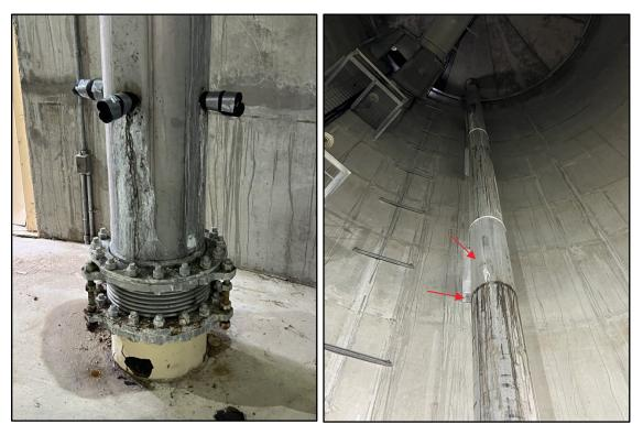
Figure 1. Site Photographs of Leaking Pipes
