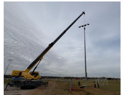
A crane installs some of the new field lighting at the Schertz Soccer Complex
