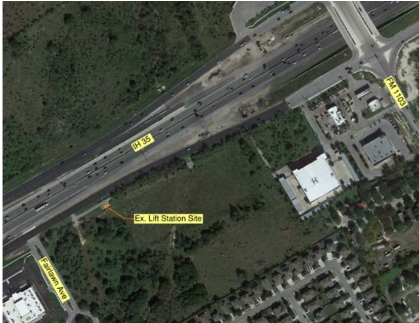
Riata Lift Station Location
