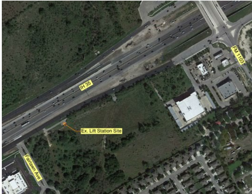
Riata Lift Station Location
