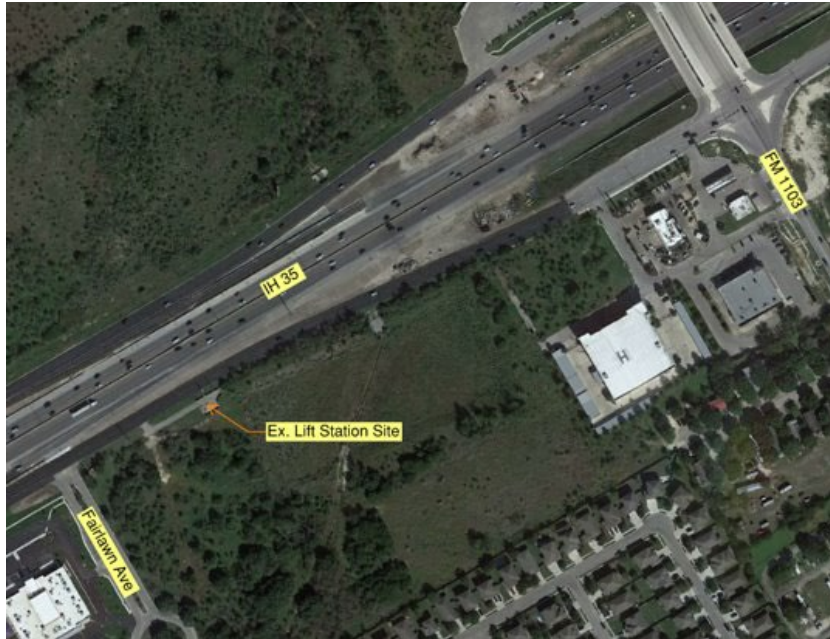
Riata Lift Station Location
