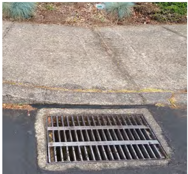
A storm water grate at the base of a curb ramp, located at the intersection of Hall Boulevard and Spruce Street.
