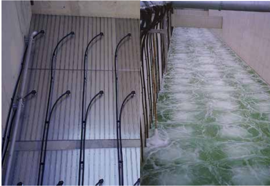
FIGURE 6 – MESSNER PANEL INSTALLED / AERATION PATTERN TEST
