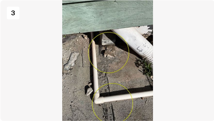
Punctures on membrane
