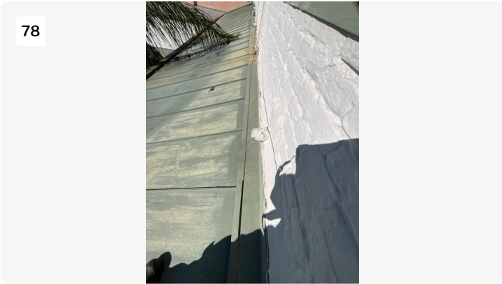
Overview of SS metal roof
