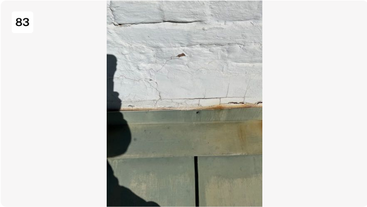
Fasteners coming undone and loose at counter flashing
