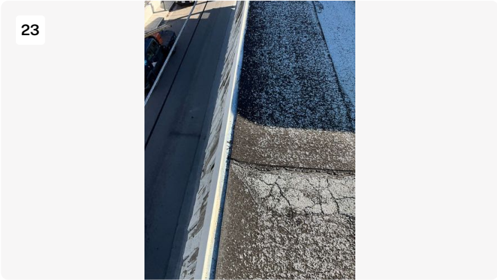
BUR membrane coming apart at roof edge/gutter transition
