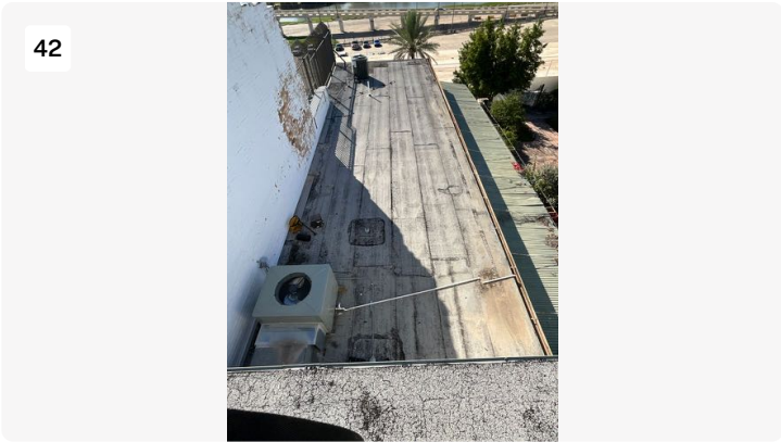
Discoloration and severe wear & tear on BUR membrane observed
