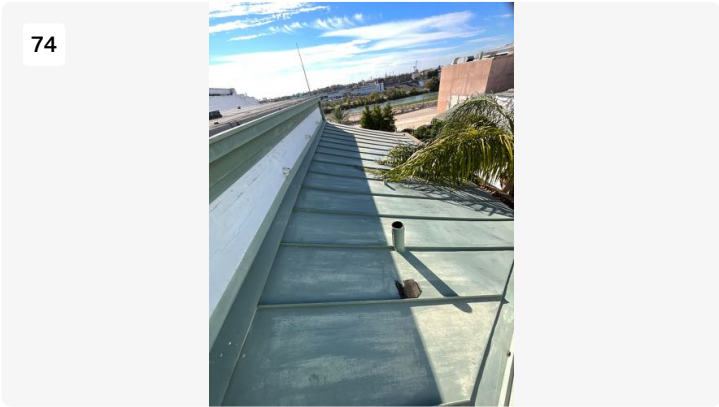
Overview of SS metal roof
