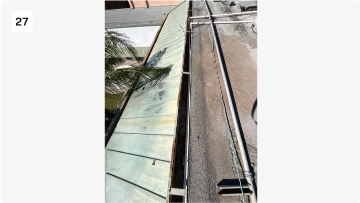
BUR membrane, gutter, and SS metal overview
