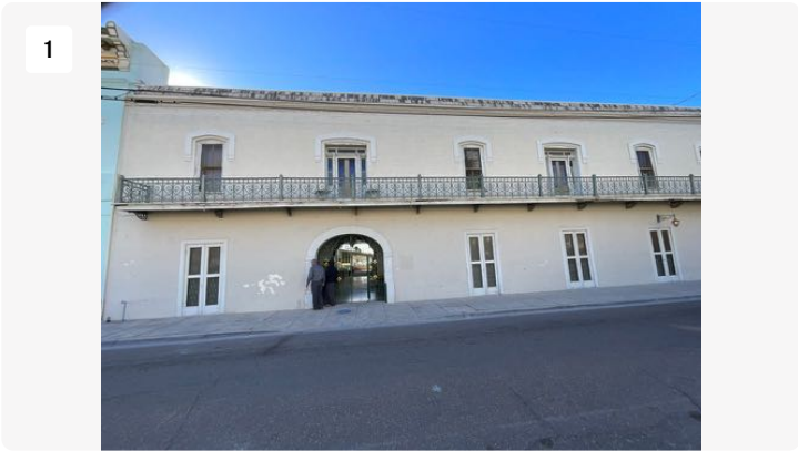
Front of building
