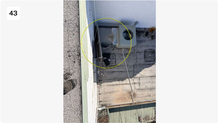
Lower section roof with window screen open
