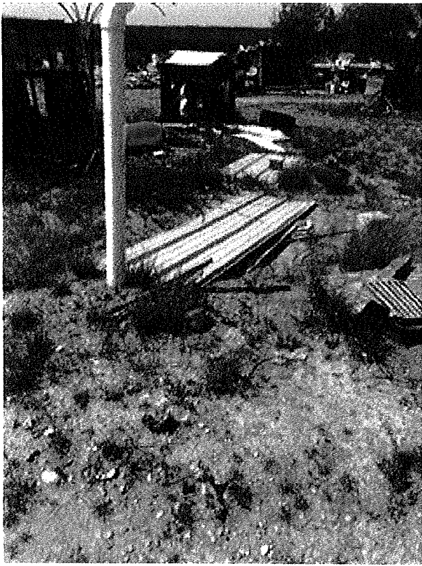
Cesspool to be eliminated with Project
