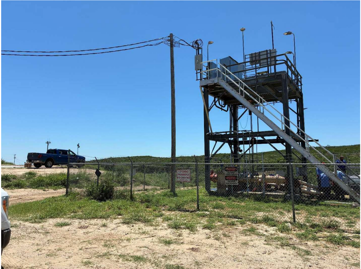
Existing conditions - fence at river intake station for rolling gate installation
