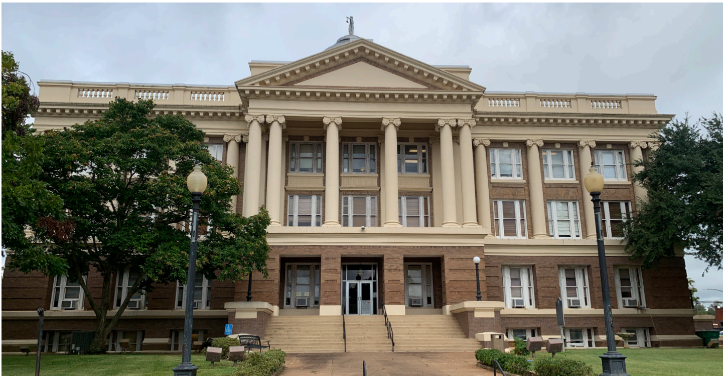
Anderson County Courthouse
