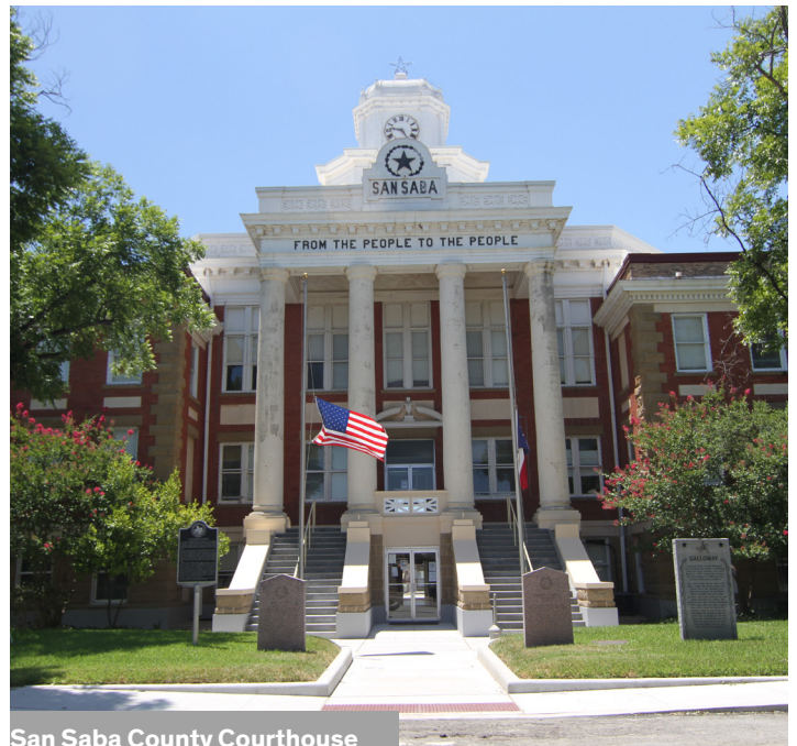
San Saba County Courthouse
