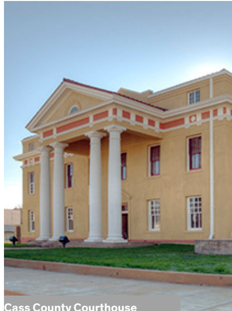
Cass County Courthouse
