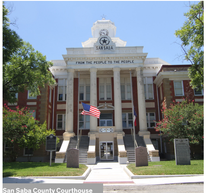
San Saba County Courthouse
